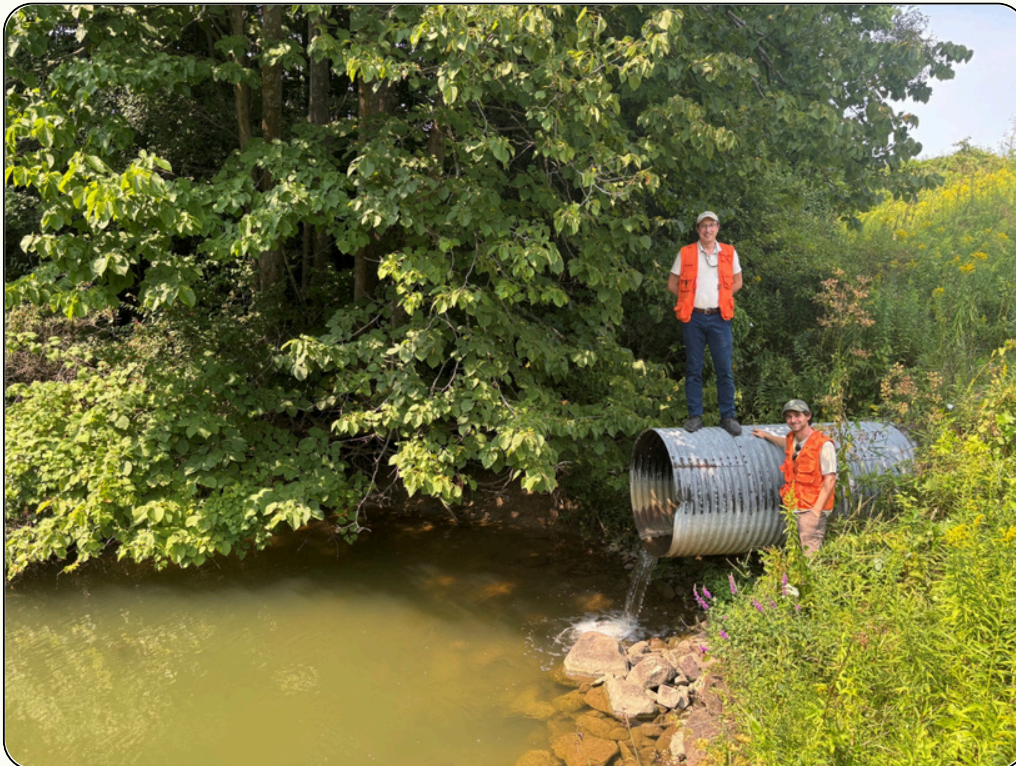
Dan Koenemann and Lucas Goldfluss conduct a site visit in Charlotte, Vermont, to assess a potential dam removal.
