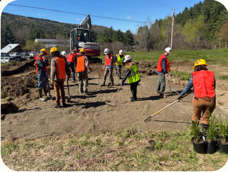
Students level out the infiltration basin prior to rain garden plant installation. Credit: Winooski NRCD
