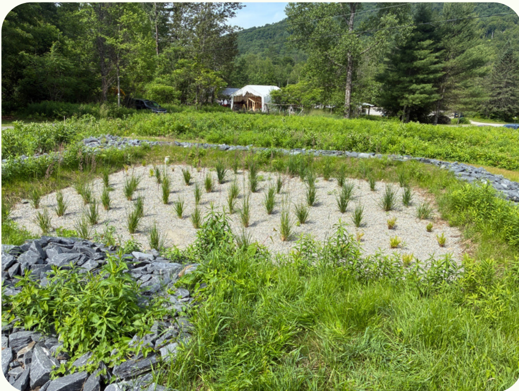
Completed infiltration basin following installation. Credit: Winooski NRCD
